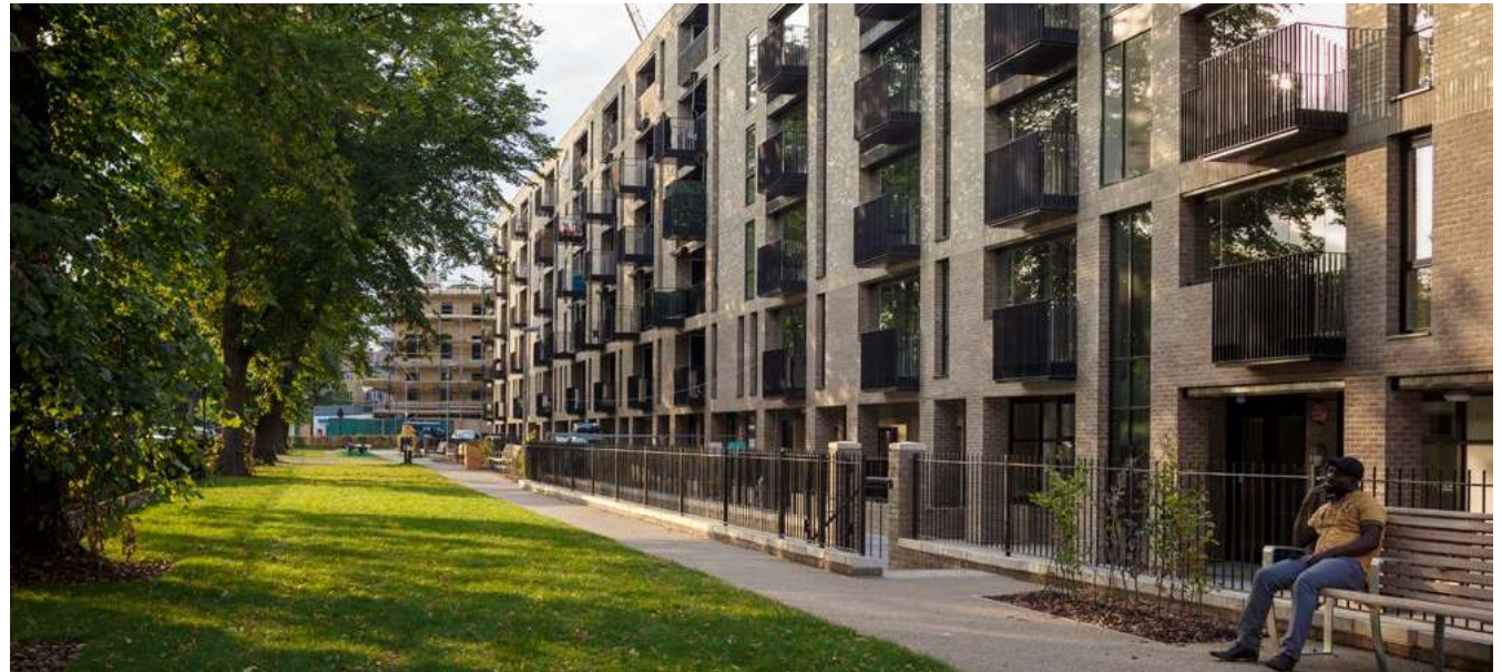
Multiple tenures including private ownership, rent, shared ownership and specialist housing groups, with no visual distinction in the facade or difference to communal entrances from the front. Buckleuch House, Clapton, London.
